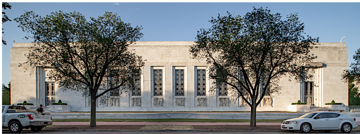
The Folger Shakespeare Library is across 2 nd Street SE, just east of the Library of Congress Adams building. The main façade of the Folger Library faces East Capitol Street NE. The white marble building is composed of modernized classical elements, which was followed by many other major buildings of the era.
